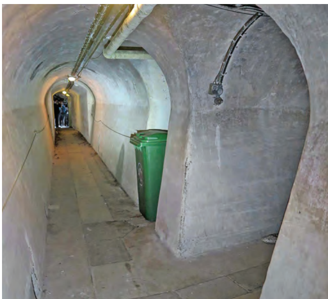
Passages beneath Dragør Fort, connecting the magazines below and gun emplacements above
